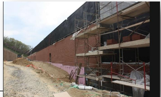
Fig. 6 Face brick facade construction
