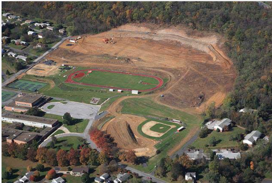
Fig.1 Aerial View of site 10-26-08
